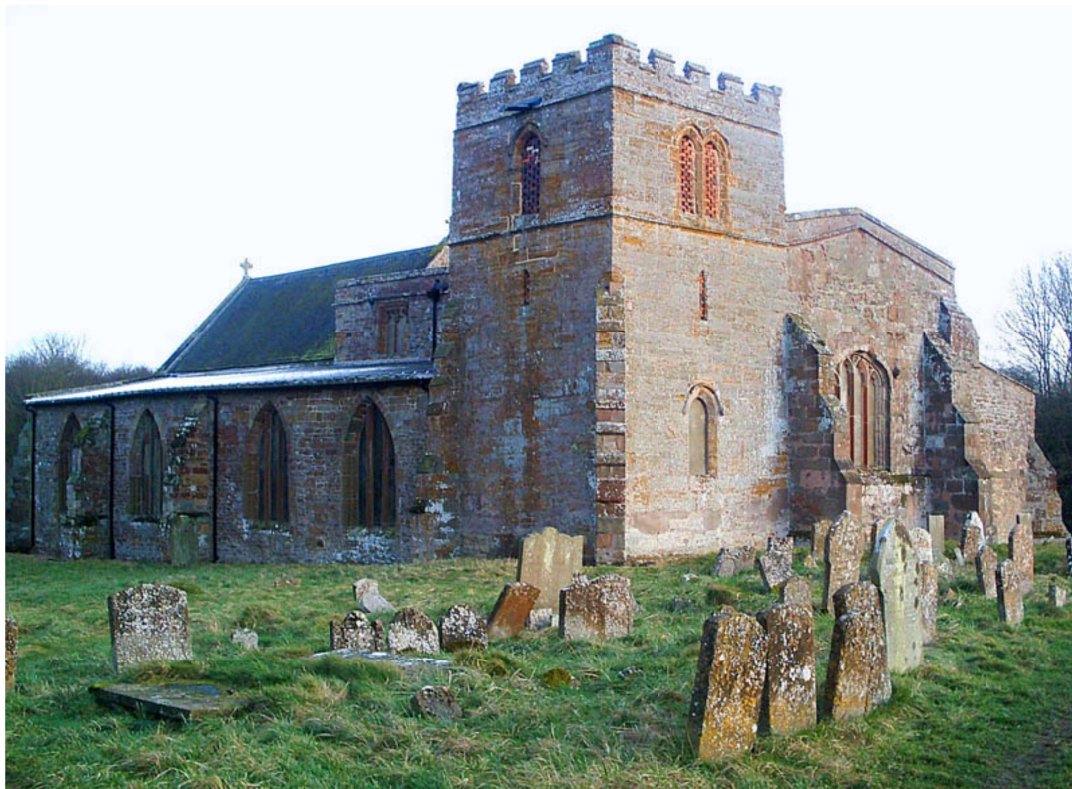
The church of Wolfhampcote standing by itself in the middle of a field
